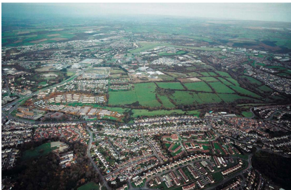
Figure I Aerial view of Derriford and Seaton
